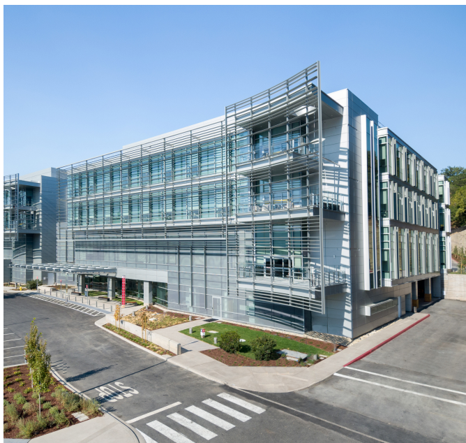
Exterior view of the Emergency Department
